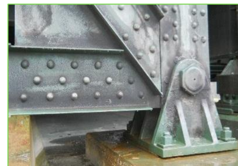
Typical Truss Bearing
