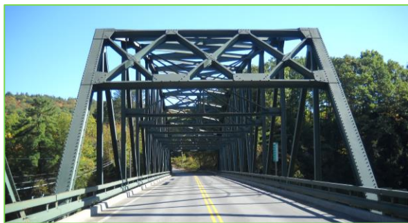
Barnet Road Bridge, Monroe, NH
